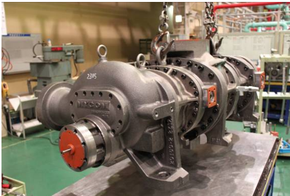
Photo 003 Lifting the Compressor
